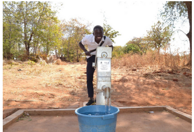
Dalireni drawing water from the rehabilitated borehole
